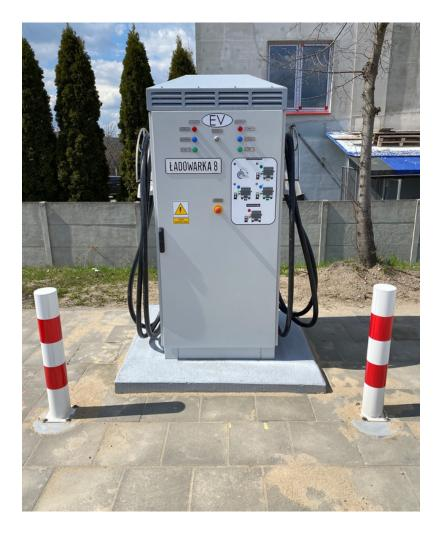
The second mode allows the user to charge a single vehicle using the full nominal voltage, i.e. 60/80/120 kW. The mode is selected automatically and is contingent on using the CCS2 connectors at the time.
