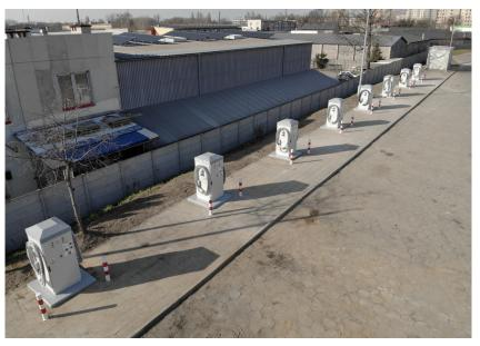
The ENI-LZ400 stationary depot charger is intended for recharging electric bus batteries.
